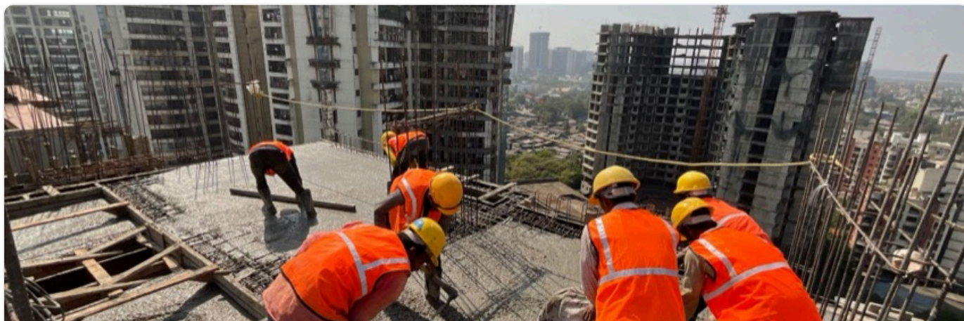
High-Rise Decks Structural pours and screeds for high-rise floors.
