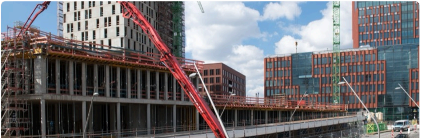
Concrete Placement Ready-mix delivery and pumped placement on site.
