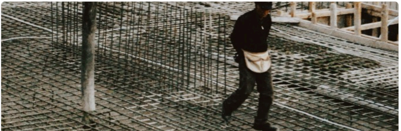
Reinforcement & Waterproofing Waterproofing systems applied before the pour.
